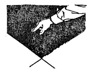
4. Start at center and place each tile on the adhesive. Make sure that first tiles are flush with the chalk lines. But each tile squarely against its neighbour, but do not slide into place. Have corners meet exactly.
